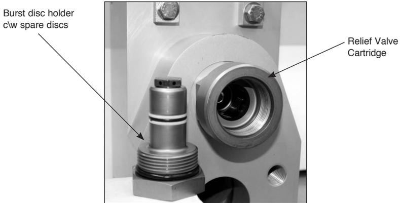
Remove the burst disc holder/catcher with a suitable socket and extract the burst discs and spacer as shown in step 2. Discard ruptured burst discs!
